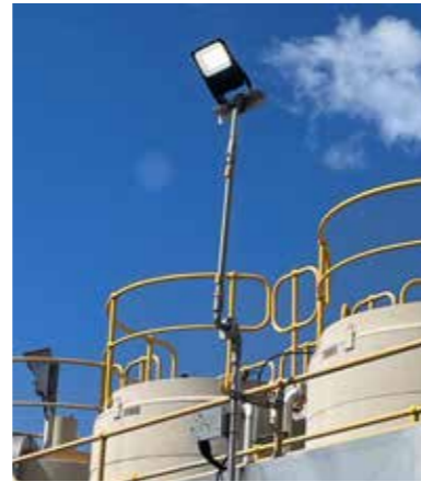
Light Poles Fully Assembled
