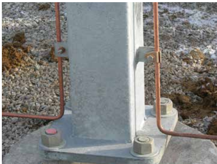
Substation earthing riser
